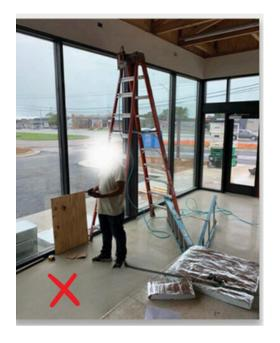
A 52-year-old finish carpenter with 20 years of experience and a co-worker were at a newly erected commercial building to install plywood panels on the ceiling. Their employer had no formal safety program. The rafters into which the plywood panels were being secured measured 11 feet, 6 inches from the concrete floor below, requiring both men to work at height.
